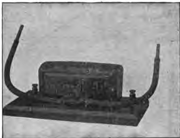
FIG. 78.—ALTERNATING-CURRENT TRANSFORMER, FERRIC MAGNETIC CIRCUIT.
