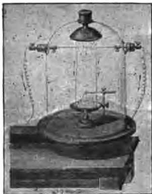
FIG. 8. TRANSMISSION OF HEAT THROUGH A VACUUM.
